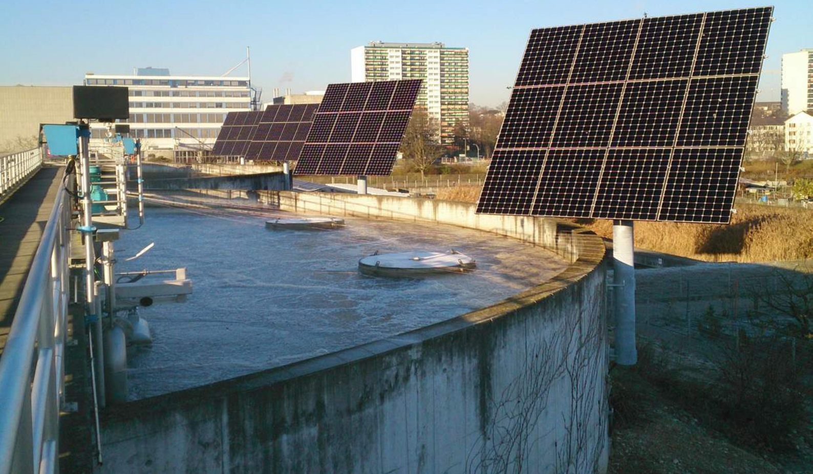
Tracking system at a wastewater treatment plant in Birsfelden in Switzerland: Degertracker 3000 HDs fitted with 12 panels each were installed.
