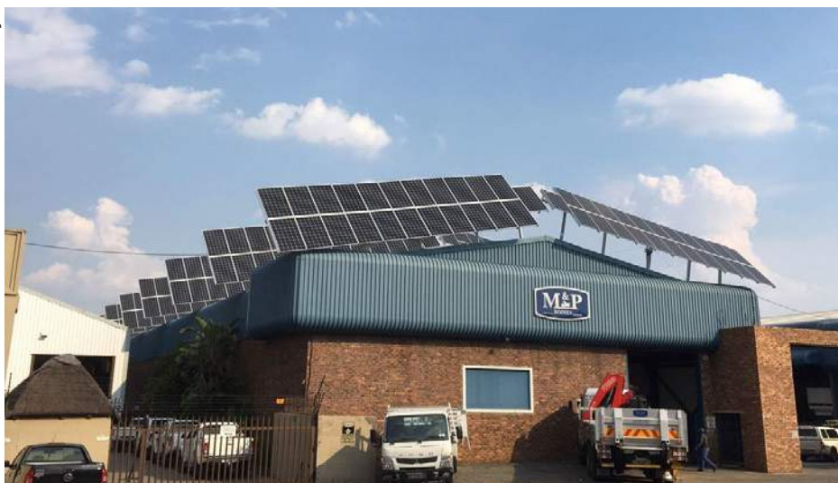
This factory in South Africa has 20 S70 trackers mounted to the steel roof.
